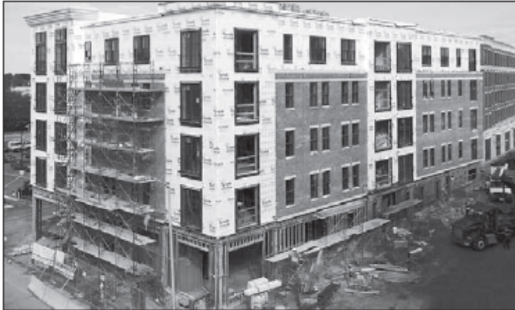
Work on the Residences at Portwalk in Portsmouth is on schedule.
